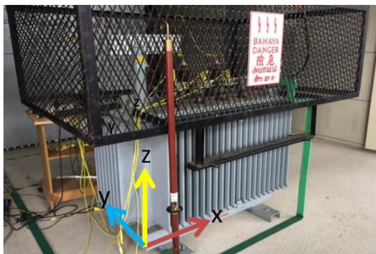
Fig. 1. Transformer at substation laboratory Universiti Malaysia Perlis, UniMAP, Malaysia
