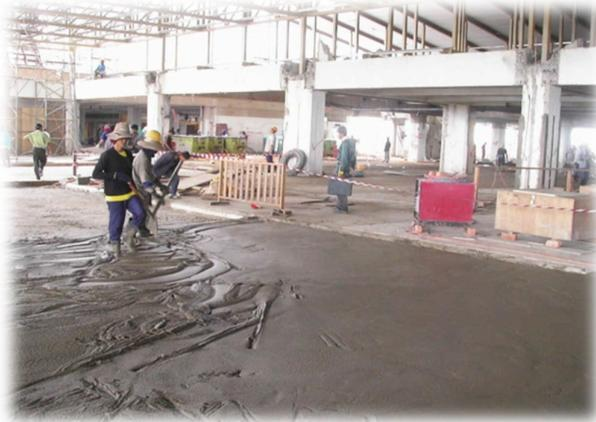
**Fig. 3.** LCM was used as underlayment and slab thickening for airport project in Malaysia ([www.drn.com.my](http://www.drn.com.my))
