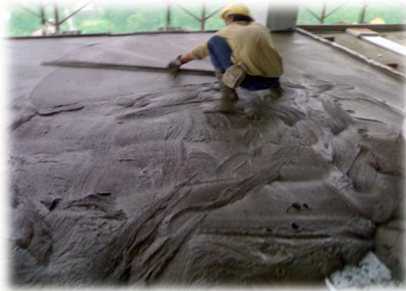
**Fig. 2.** LCM was poured in sections to prevent loss in density and reduce shrinkage problems in slabs for UEM Building Kuala Lumpur ([www.drn.com.my](http://www.drn.com.my))
