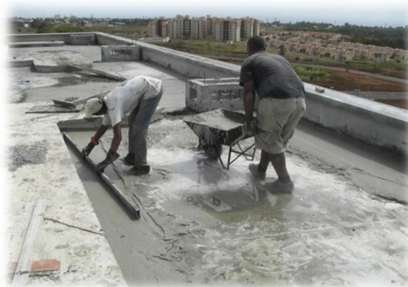
**Fig. 1.** LCM insulation screed was utilized to offer thermal protection for a multi-storey building in Mauritius ([www.drn.com.my](http://www.drn.com.my))
