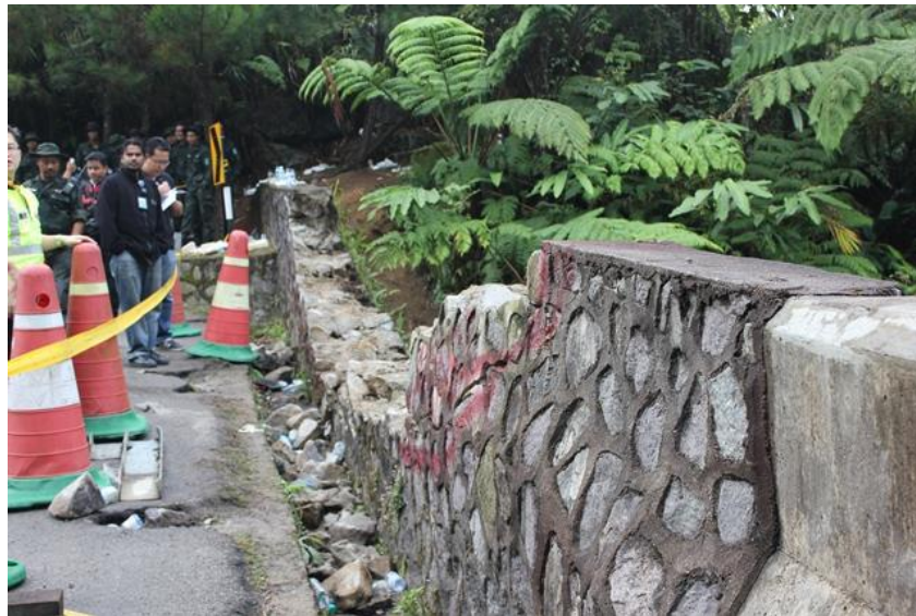
Fig. 2. Damaged guardrail and rubble wall at the crash site
