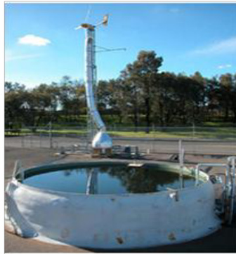
Figure 7-3: Bundoora Chimney Solar Pond Combination [5]
